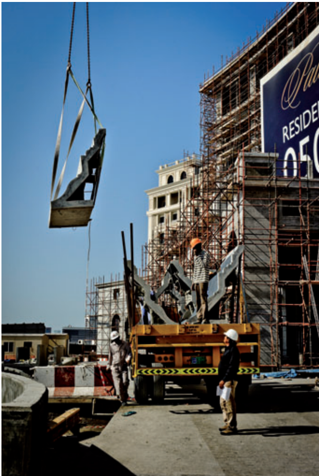
Lifting of a GRC cornice in the Palazzo Versace
