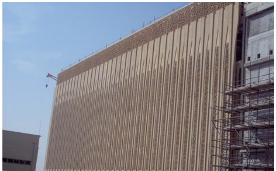
Large size panels hanged on the structure of the Dubai Mall
