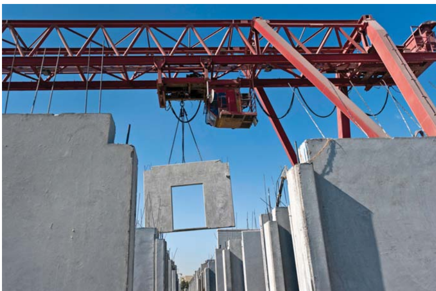
Precast wall panel storage.
