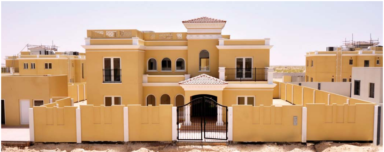
Completed villa with boundary wall and GRC decorative elements.
