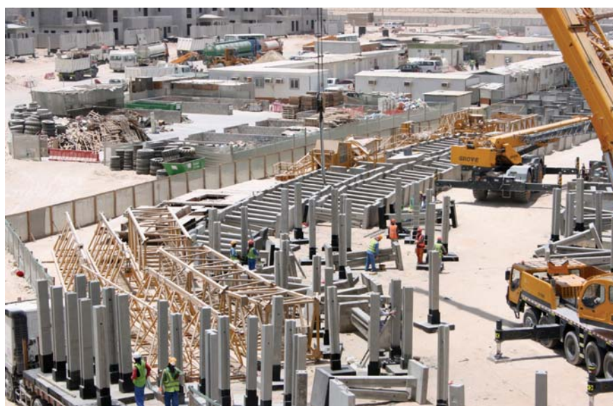
On-site semi-mobile factory.
