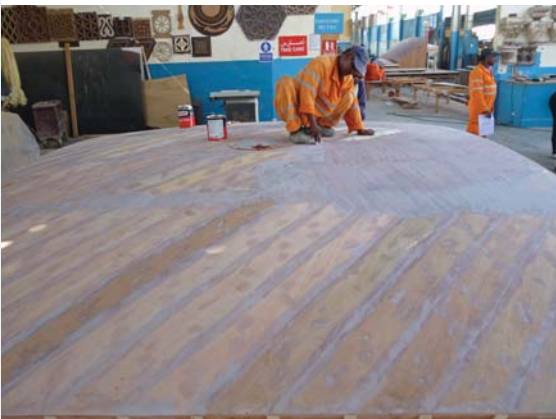
Production of a wooden counter-mould for GRC dome segments.
