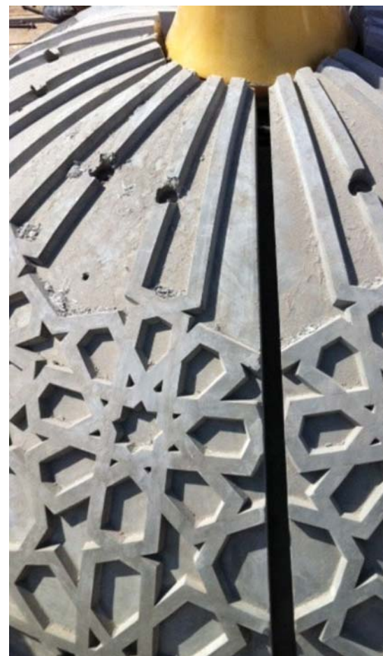
Right: Patterned dome segments that will be mechanically fixed.
