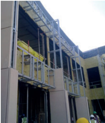
Fixing GFRP elements on the steel envelope.
