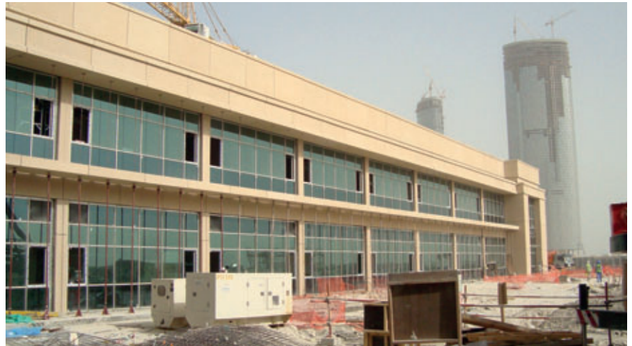
Windows sunk from the façade
