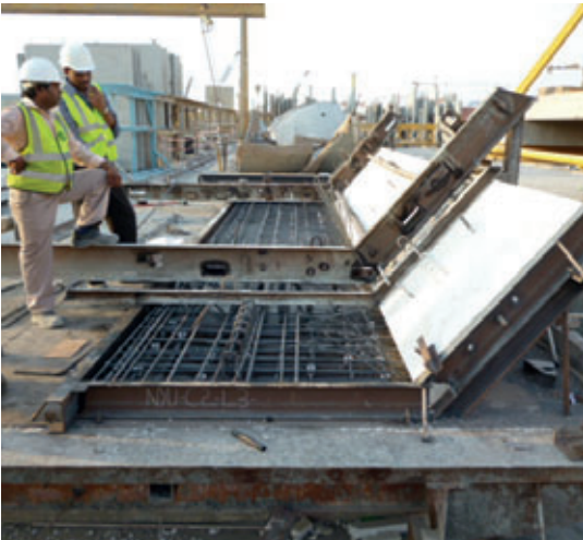
Preparation for casting of the second side of V shaped elements
