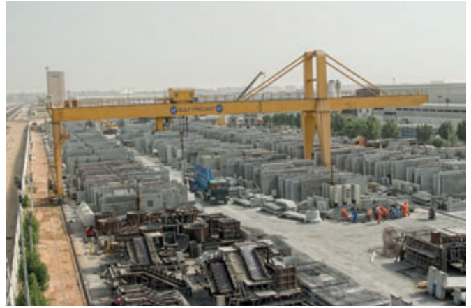
A Precast Factory stockyard
