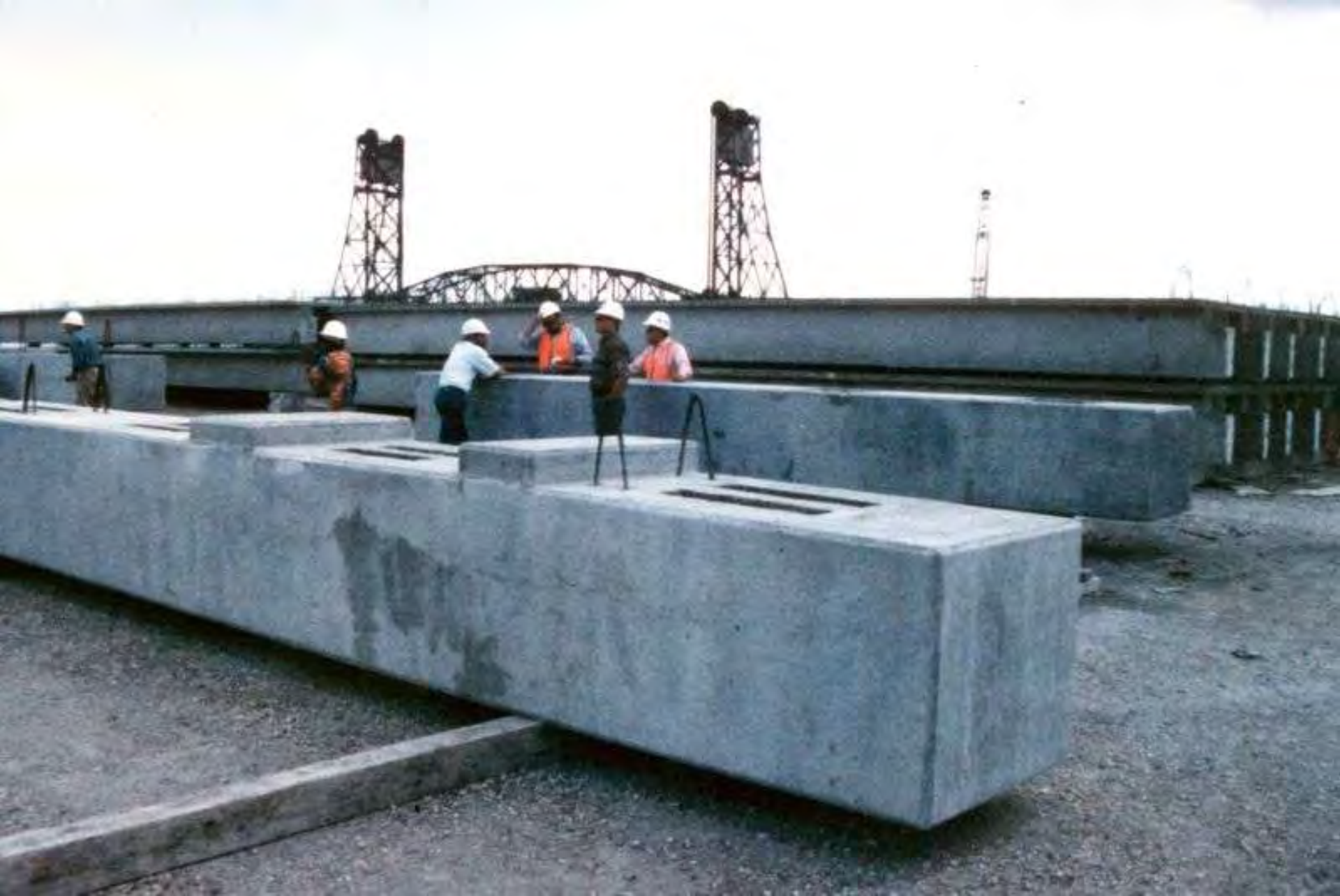
Redfish Bay Bridge-Texas, Precast Pier Caps
