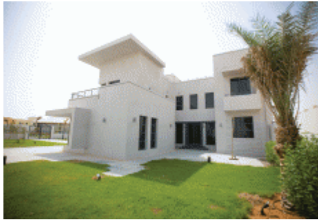
Gulf Precast is building 2,000 villas at Al Falah in Abu Dhabi.
