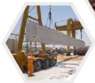
6. Lifting and storage
