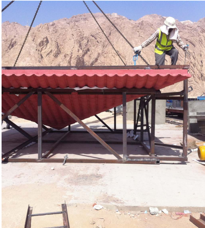
On-Site Semi-mobile production plant in Al Ain Emirati housing complex, producing GRC slopped roof too large to transport by roads
