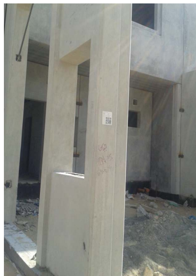
Bar coded Precast Panels after erection in Al Falah Community housing complex.
