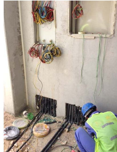
MEP inserts imbedded in the Precast Elements in Al Ain Emirati housing complex
