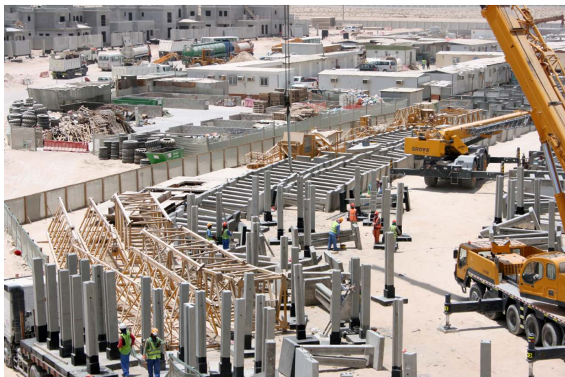
On-Site Semi-mobile production plant in Al Falah community development, producing columns for Boundary Walls
