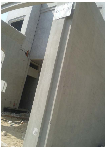
Bar coded Precast Panels after erection in Al Falah Community housing complex.
