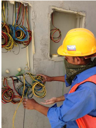
MEP inserts imbedded in the Precast Elements in Al Ain Emirati housing complex
