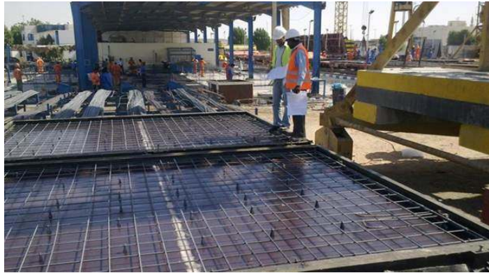
Inspection before Casting
