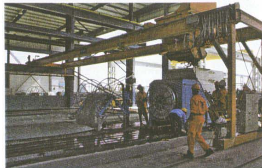
Fig. 4 The half portals automatically follow the forward-traveling production machine and each half-portal automatically activates the respective bucket rail system.
