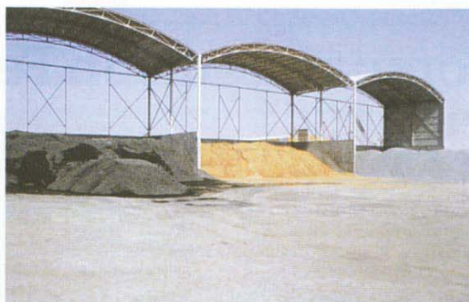
Fig. 1 Storage of aggregates, cements and other raw materials at Gulf Precast.
