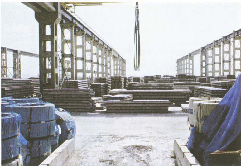
g. 7 Storage yard for the precast hollowcore slabs.
