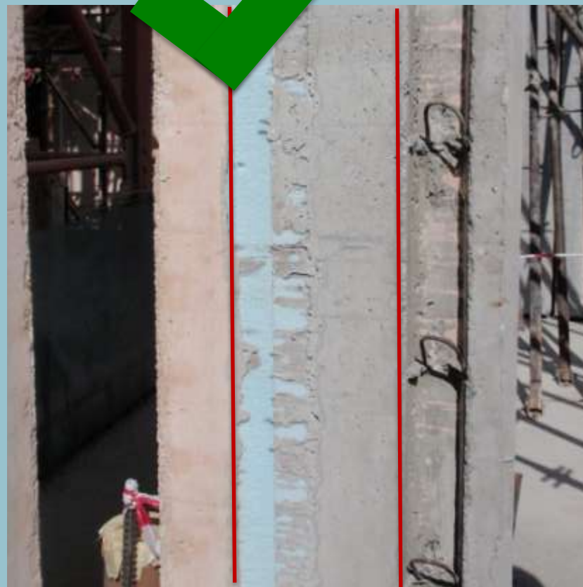
Insulation full length of wall
