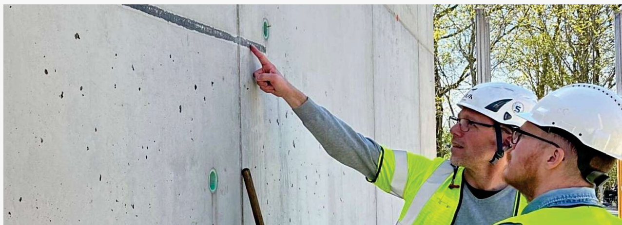
Gripcon used in NCC project for mounting kitchens and wardrobes
